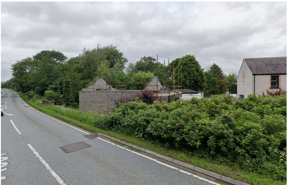
Figure 5. Construction of garage/workshop at 'The Old Steading'.
